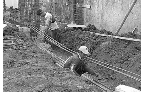
Figure 7. Sloof Reinforcement Installation Work
